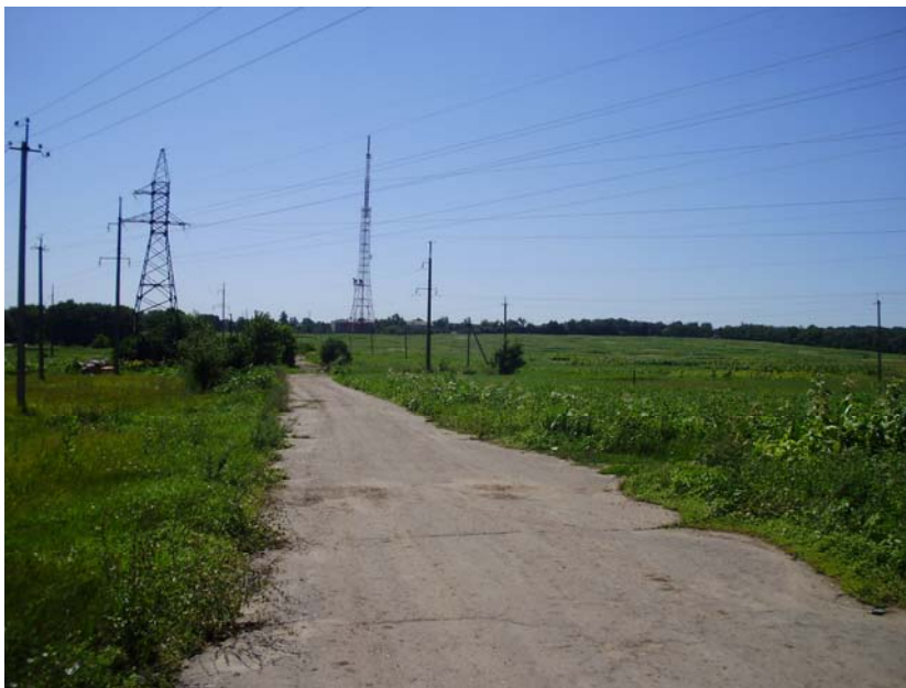
Small site road, North-South direction. Low and high voltage air cables. Broadcasting tower in the background
